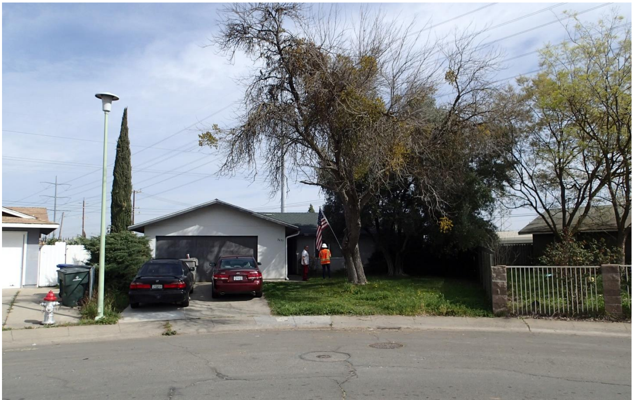
Photo 1: View of the Meza property facing northeast from Fallis Circle. The existing residential structure would be demolished and an access road extended from Fallis Circle to the PG&E valve lot behind the house.
